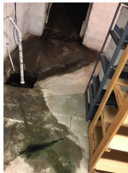
Standing water, mold and floor cracks in basement archival storage
