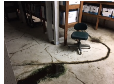
Standing water, mold and floor cracks in basement archival storage
